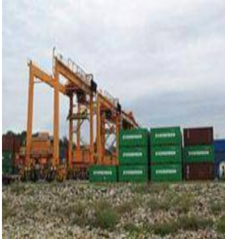
Fig6.6: Containers Yard with rubber tyre
